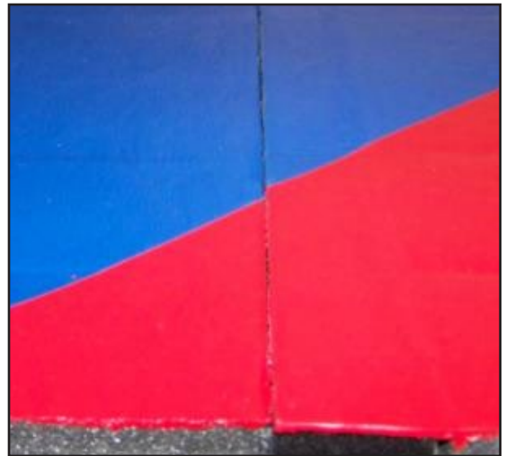
Improperly setup FLEXI-Connect ® mat with overlapping seam.
